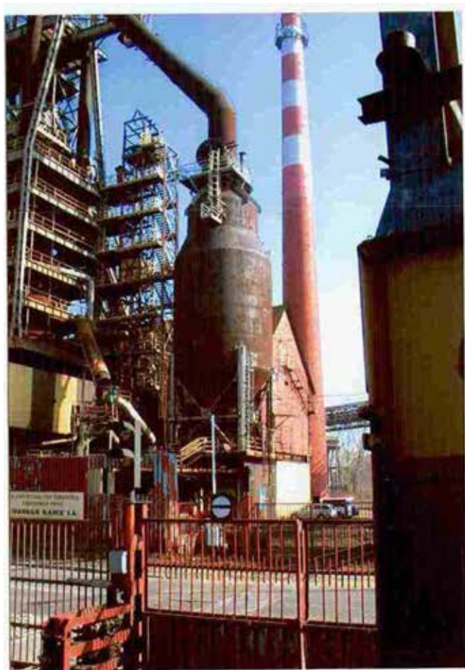
View of the passenger and cargo lift tower (between the static dust catcher and the blast furnace) to the south-west.
