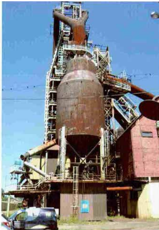
VIEW OF THE BLAST FURNACE "A" COMPOUND FROM THE SOUTH IN THE FOREGROUND, THERE IS THE STATIC DUST CATCHER
