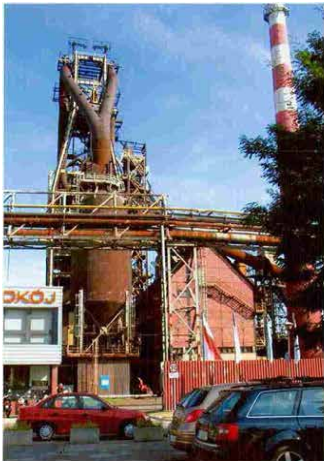
VIEW OF THE BLAST FURNACE "A" COMPOUND FROM THE SOUTH IN THE FOREGROUND, THERE IS THE STATIC DUST CATCHER AND THE BUILDING HOUSING THE PUMP ROOM, FILTERS AND CONVERTER
